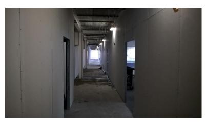
Works continue in closing up the façade which has allowed our internal fit out operations to begin. As can be seen from the photograph opposite the internal walls are now being formed (picture from 1<sup>st</sup> floor corridor) Brickwork to external walls has also started. We have one large concrete pour remaining. This is confirmed for 22<sup>nd</sup> February.
