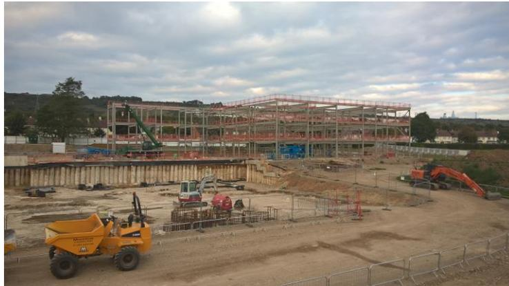
The structural steel frame installation is now well progressed, as can be seen from the photo adjacent. As the steel frame continues we will begin to install the floors and staircases within the structure. These are pre-cast concrete units which are delivered to site in sections for installation. This reduces the amount of ready mixed concrete that we have to place on site, and the associated deliveries.
